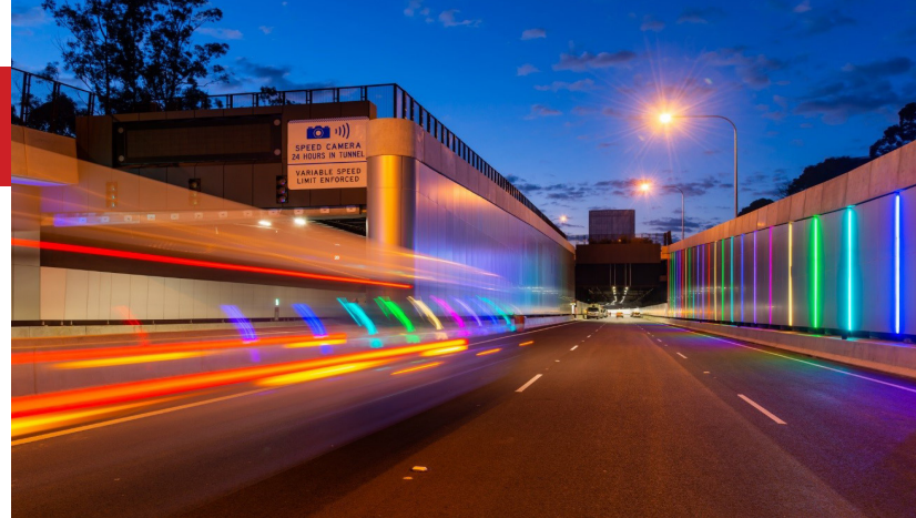
M4 East Tunnel Entrance Photo provided courtesy of Transurban
